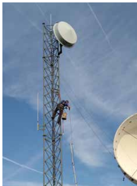
Bob Isby, K2RHI, raises the new 220 mhz repeater antenna on the HVCC tower
